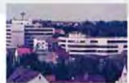
1980: Company Construction starts on adidas administration building II in Herzogenaurach
